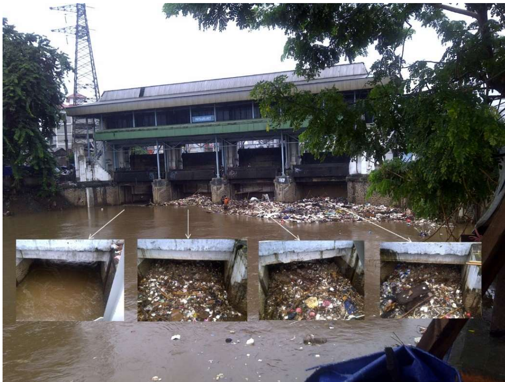
Fig. 2.5 Trash accumulation situations at the Karet gate after the flood event (Photos provided by Deltares)
