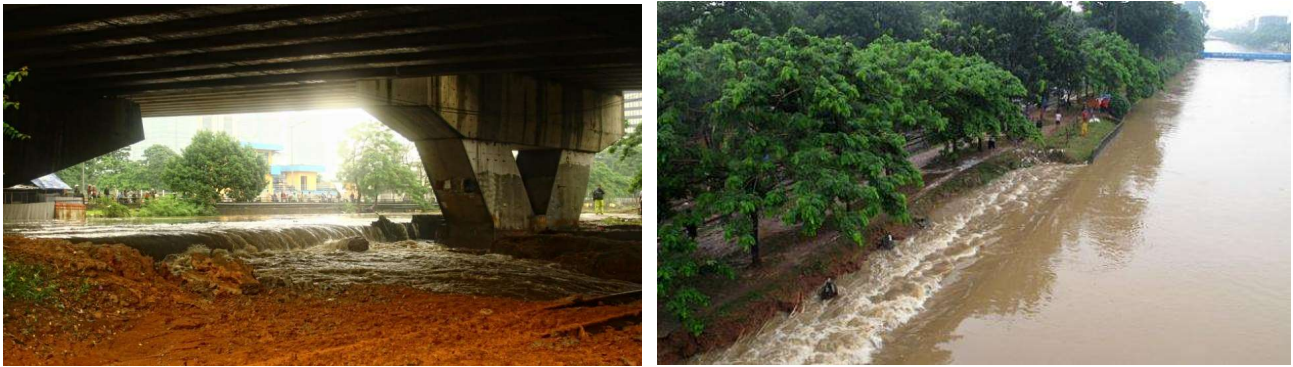
Fig. 2.4 Overtopping situations at the section of embankment along the west drainage canal (Photos provided by BNPB)
